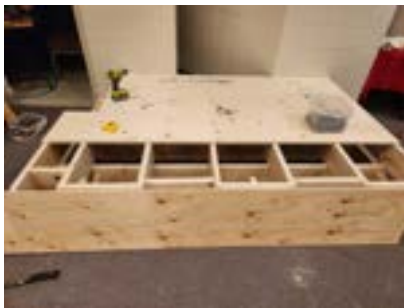
The flooring being installed.
