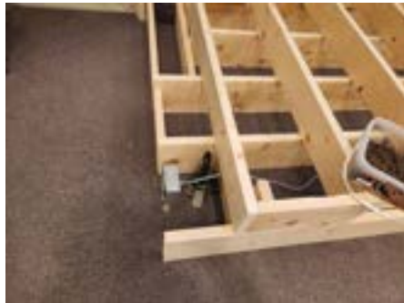
The Lower Framework and Signal Feed Conduit
